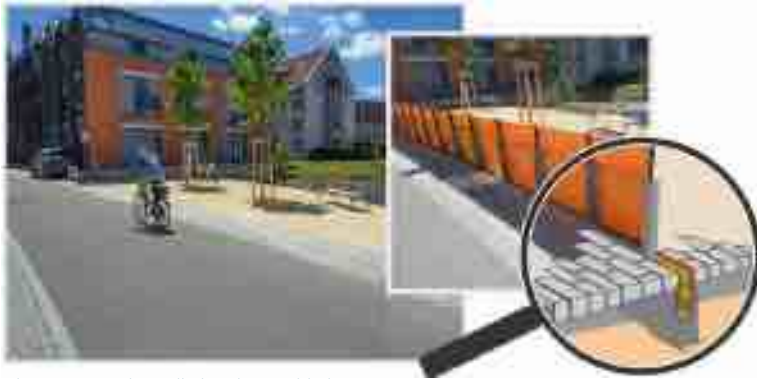
The AquaWand installed and assembled.
