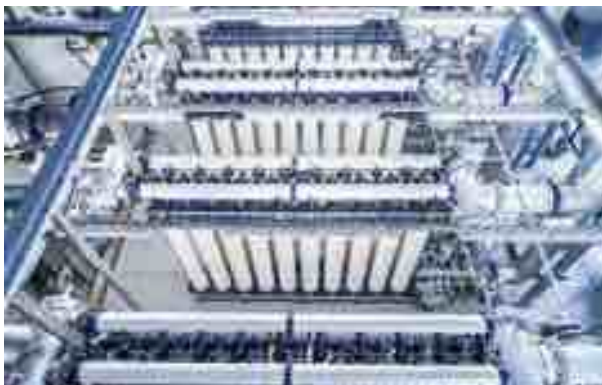
Ultrafiltration plant for water treatment (T-Rack® system)
